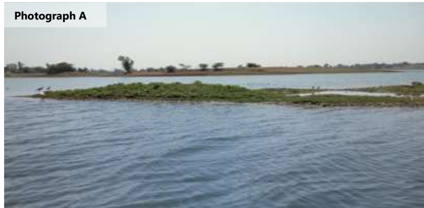
Photograph A: South-east side of the Patadungri dam wall (427086 mE, 2512620.1 mN) showing an isolated island within Patadungri Reservoir
