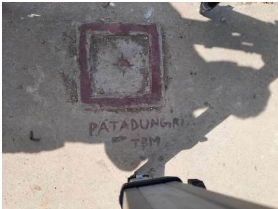
Figure 3.1: Client Supplied Benchmark (Patadungri-TBM)
